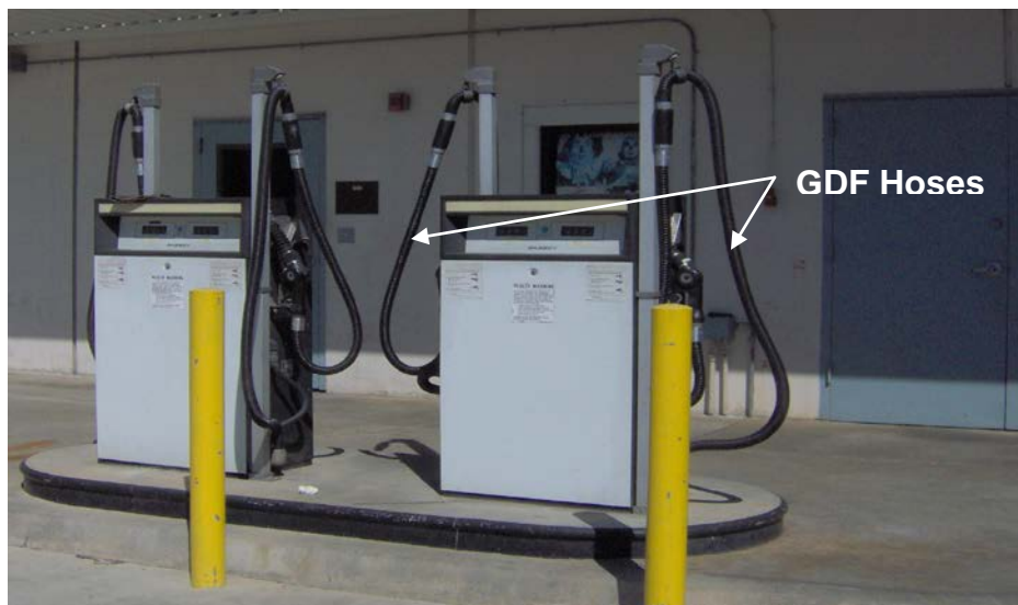
Figure II-2. GDF Fuel Hoses
