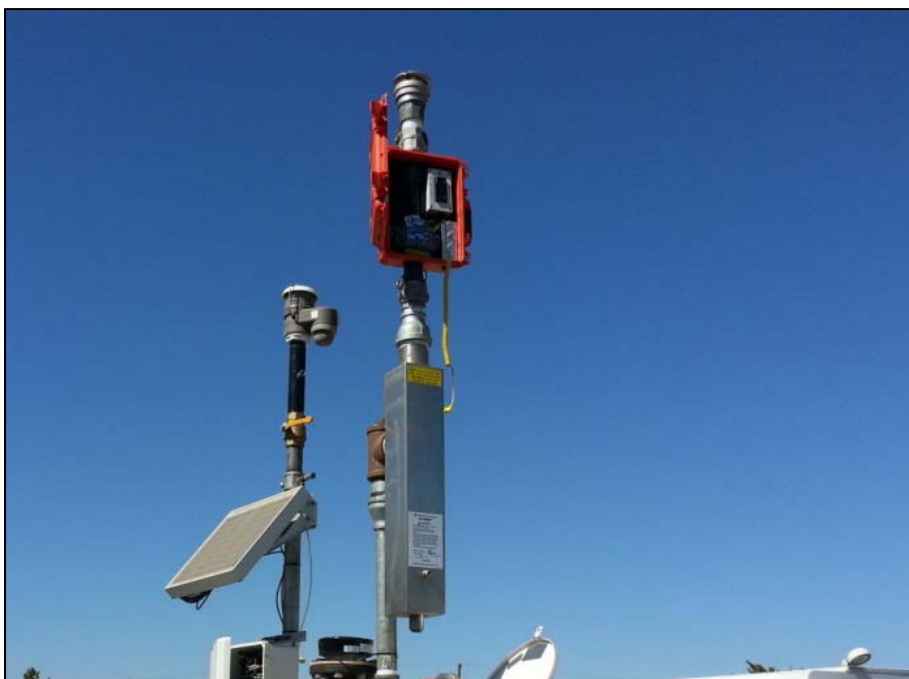
Figure 1B: Typical Installation of PV-Zero on Single-Wall AST (with Vent Pipe Volume Meter)
