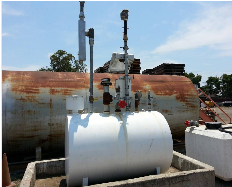
Figure 1A: Typical Installation of PV-Zero on Single-Wall AST
