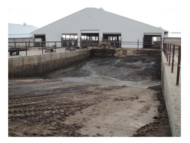
•A small, usually concrete-lined structure used to regulate flow of flushed manure prior use of a mechanical separator
