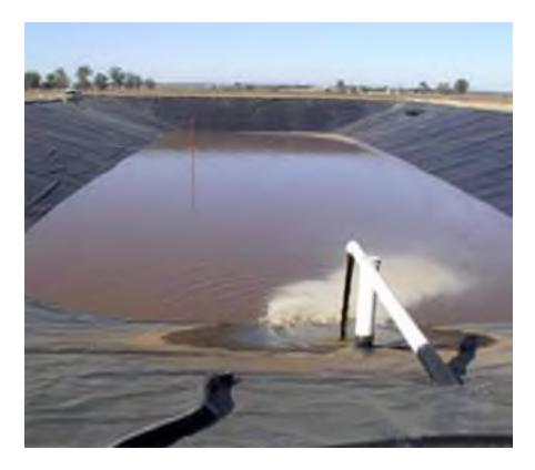
•A large retention pond intended to collect water and manure as it is flushed. The supernatant (water from the upper layers of the pond) may be recycled to use as flush water in housing areas but not milking barns.
