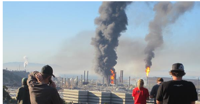
Above: Commuters step out of their cars to take pictures of the fire raging within the Chevron oil refinery on Aug. 6, 2012, found by the US Chemical Safety Board to be the result of repeated failures of Chevron to fix known metal thinning, and due to increases in corrosive sulfur in crude oil (which Chevron had tried to discount during environmental review of an expansion). This explosion narrowly missed killing 19 workers, and sent thousands of residents fleeing the black clouds.
