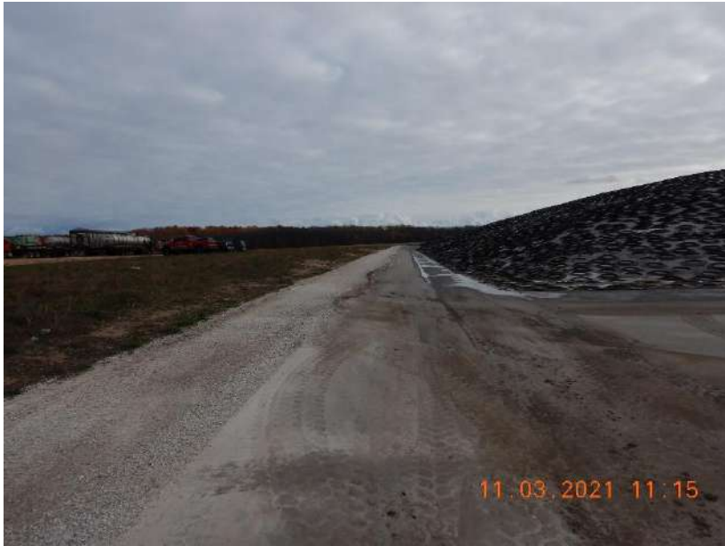
Photo 98. The north side of the feed storage area at Site 2. The pitch in the concrete prevents runoff from leaving the north side of the feed storage area. This photo was taken facing west.
