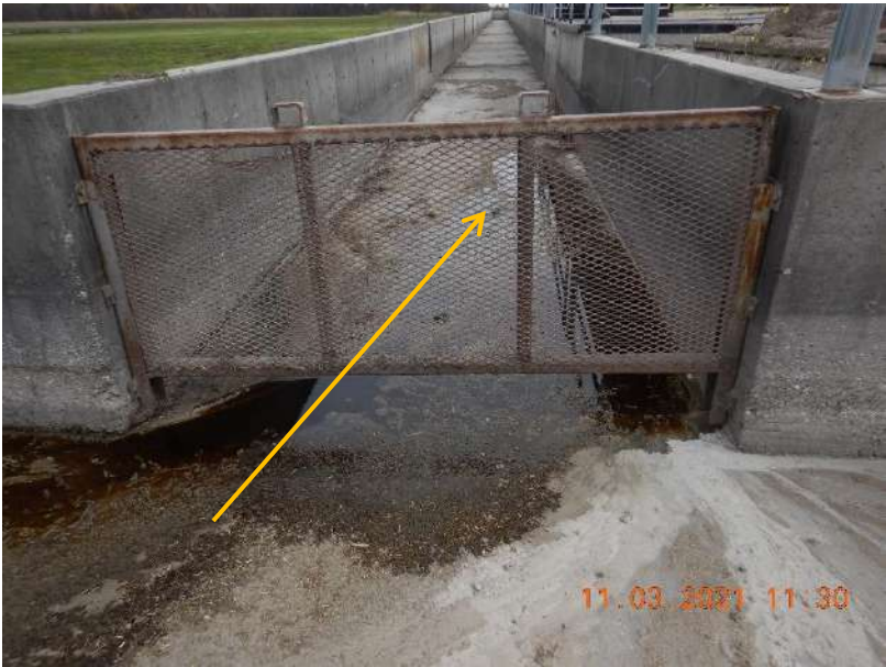
Photo 108. The concrete spreader bar that evenly distributes runoff across the VTA. The VTA is currently not being used to treat runoff. This photo was taken facing east.
