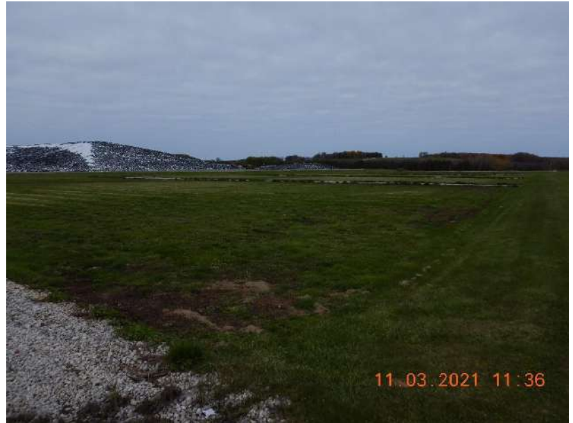
Photo 120. An earthen berm located on the east side of the VTA. The berm prevents runoff from leaving the VTA. This photo was taken facing north.
