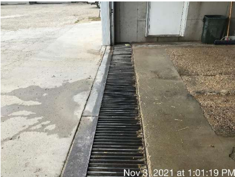
Photo 86. The flume system that captures process wastewater from the machine-washing area.
