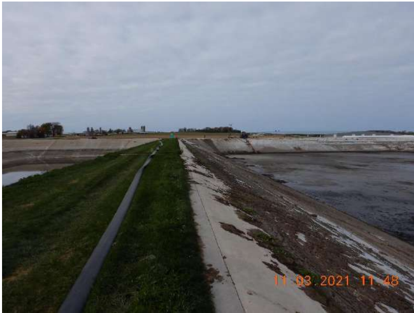
Photo 35. The concrete weir that connects WSF 5 and WSF 6. The weir is used as an emergency transfer system to allow manure to be transferred between the two WSFs. This photo was taken from WSF 5.
