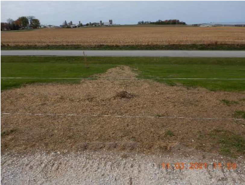
Photo 156. A grassed swale located between the southern feed storage area and WSF 2 at Site 1. The swale conveys stormwater through the production site.
