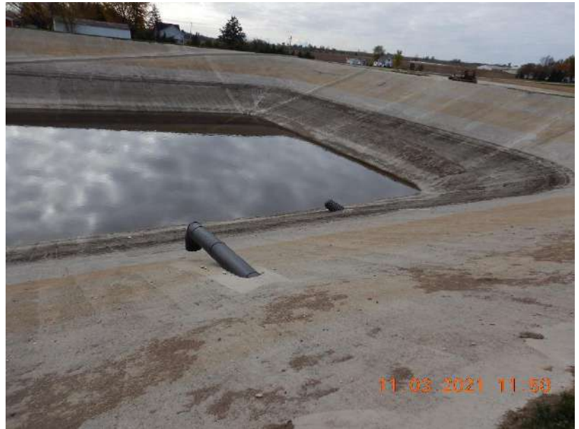
Photo 33. The permanent markers present within WSF 6 at Site 2. The markers do not account for the 25-year, 24-hour runoff collected from the feed storage area.
