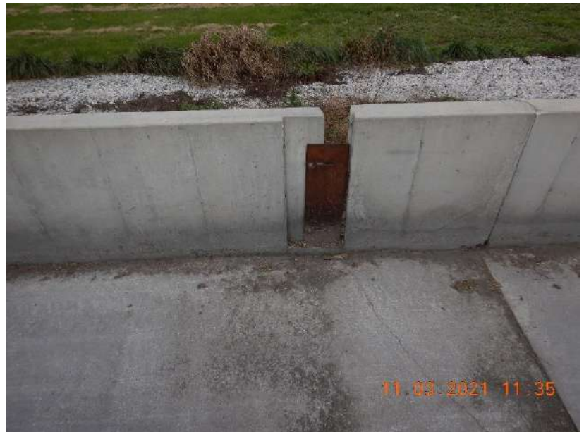
Photo 111. The area where runoff enters the collection inlet. The flow path of runoff is represented by the yellow arrows.
