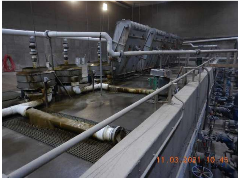
Photo 51. Pumps that transfer liquid manure through the flume system in the freestall barn at Site 2 to flush the flumes while pens are being cleaned.
