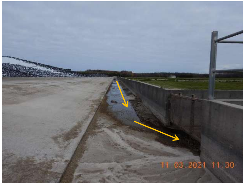
Photo 107. The metal grate that captures solids and prevents the solids from entering the collection system. The flow path of runoff is represented by the yellow arrow.
