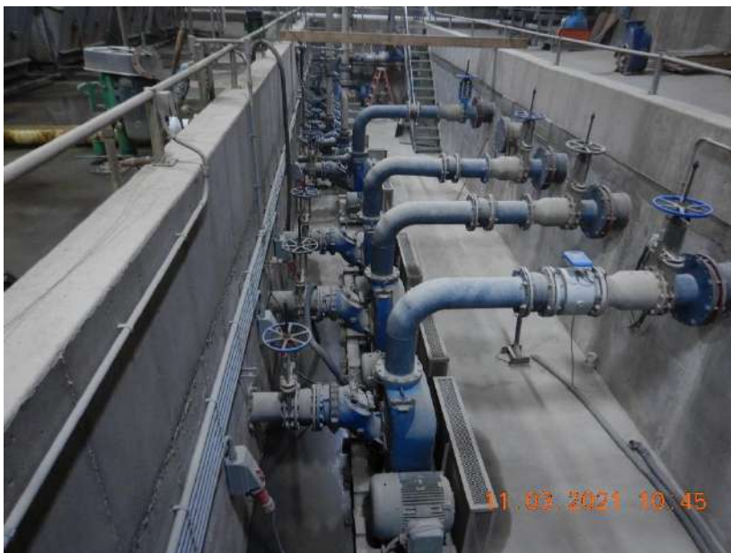
Photo 51. Pumps that transfer liquid manure through the flume system in the freestall barn at Site 2 to flush the flumes while pens are being cleaned.
