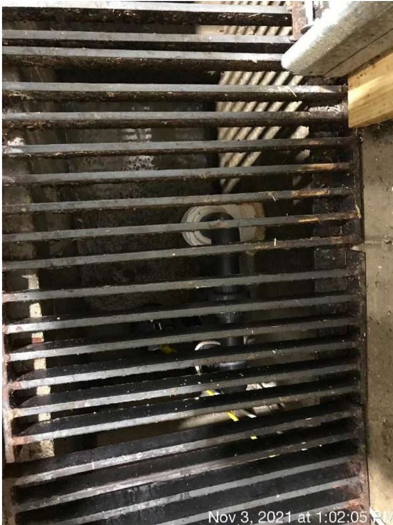
Photo 87. The pump that transfers process wastewater from the machine-washing area to the manure transfer system.
