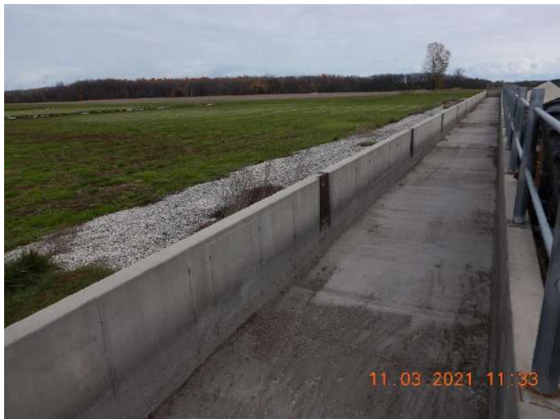
Photo 108. The concrete spreader bar that evenly distributes runoff across the VTA. The VTA is currently not being used to treat runoff. This photo was taken facing east.
