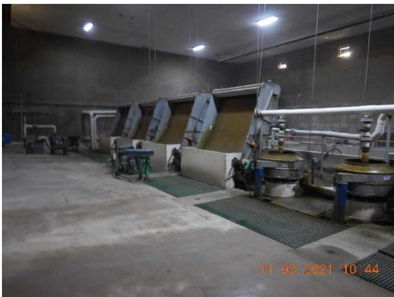
Photo 48. The sand separation building at Site 2. Sand bedding that enters the manure transfer system in the freestall barn at Site 2 is removed from the manure, cleaned, and stored in this location until it is reused for bedding.
