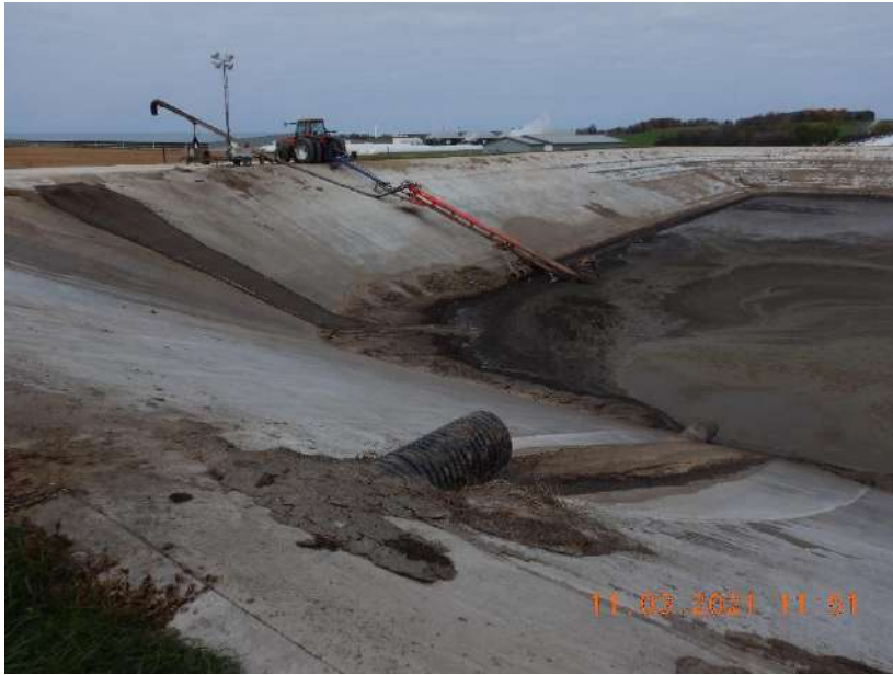
Photo 26. One transfer pipe that allows waste to be transferred from WSF 6 to WSF 5. This photo was taken facing north.
