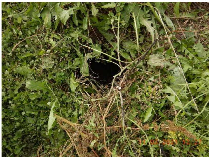
Photo 18. Animal burrowing present in the berm around WSF 2.
