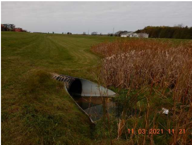
Photo 151. A stormwater culvert that discharges clean water to the detention pond pictured in Photo 150. This photo was taken facing west.
