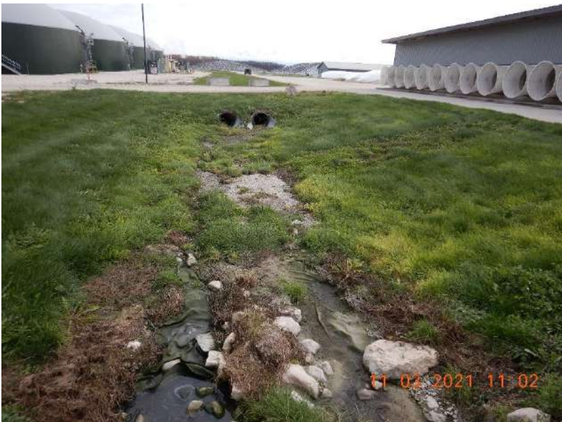
Photo 145. A grassed swale on the north side of the freestall barn at Site 2 that is used to convey stormwater through the production site.
