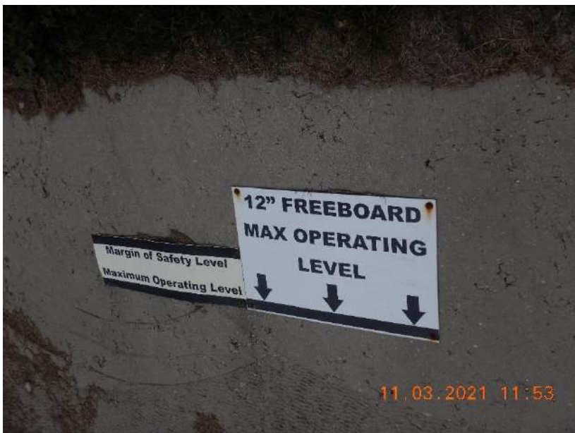
Photo 33. The permanent markers present within WSF 6 at Site 2. The markers do not account for the 25-year, 24-hour runoff collected from the feed storage area.
