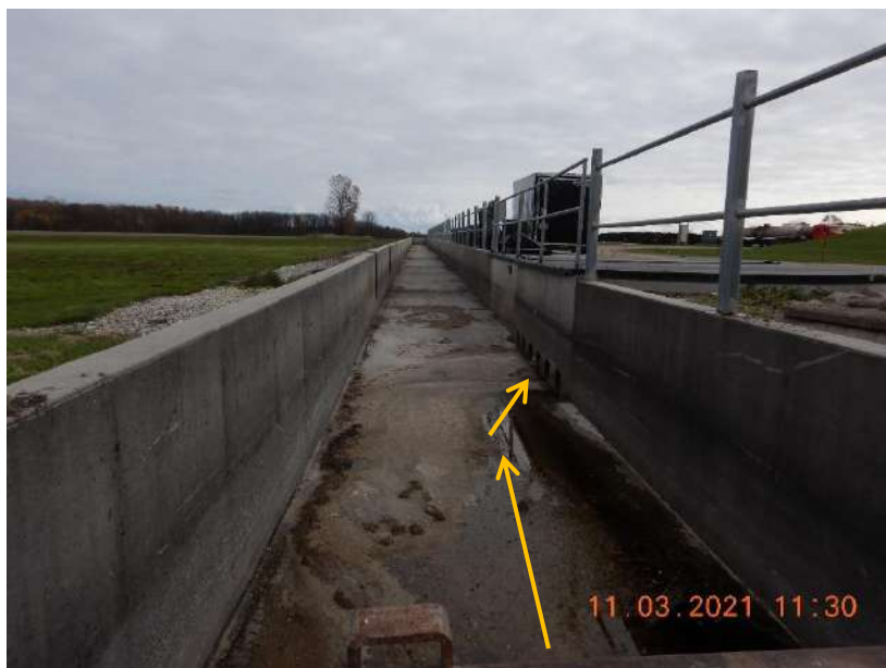
Photo 111. The area where runoff enters the collection inlet. The flow path of runoff is represented by the yellow arrows.
