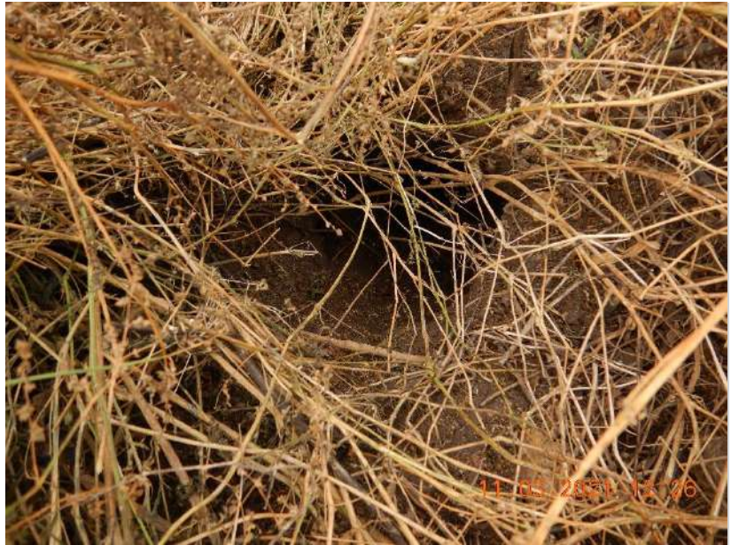
Photo 18. Animal burrowing present in the berm around WSF 2.
