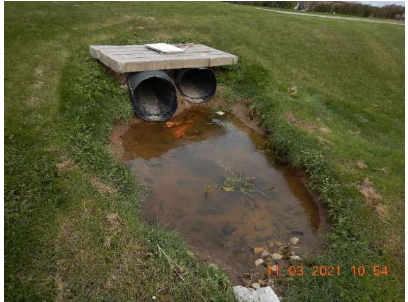
Photo 145. A grassed swale on the north side of the freestall barn at Site 2 that is used to convey stormwater through the production site.
