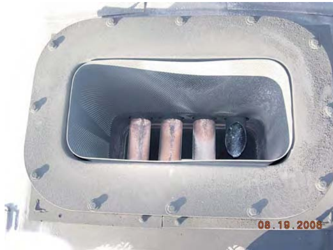
Figure 4: View into the Dash 8 exhaust stack, showing the crankcase vent and air filter suction tubes
