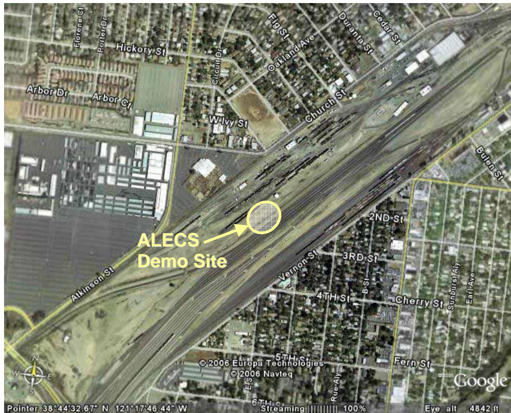
Figure 19. Aerial View of the Site Where the ALECS was Installed
