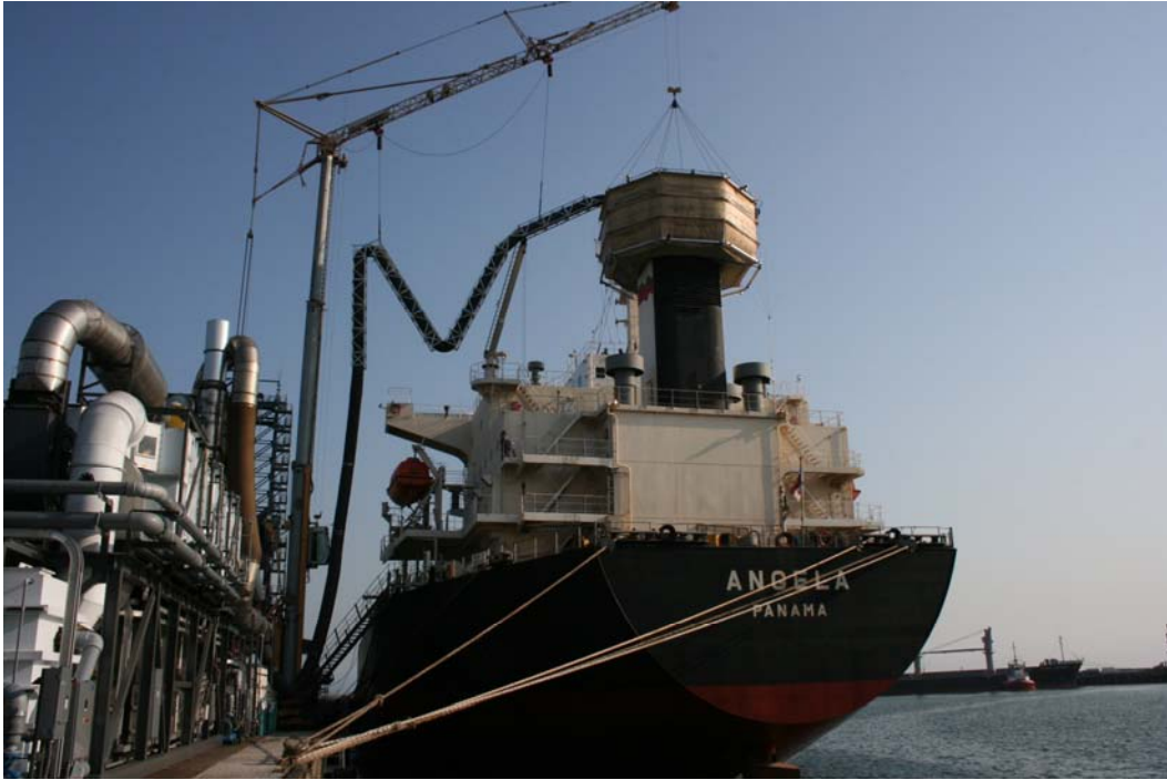
Figure 15. Emission Capture System Attached to the Angela
