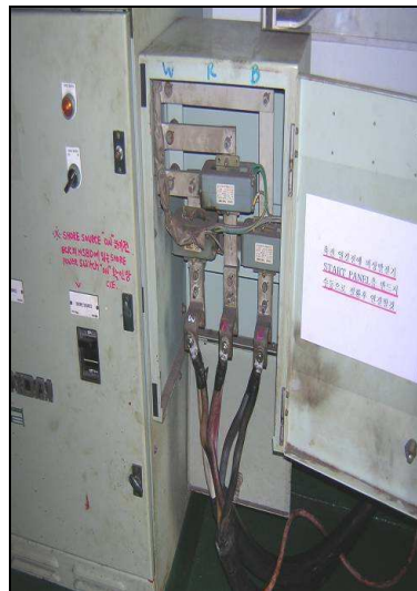
Figure IV-8: Shore power connection on the Pacific Success at the USS POSCO facility
