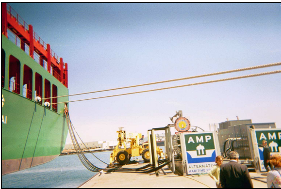
Figure IV-1: Shore Power Provided via a Barge at China Shipping
