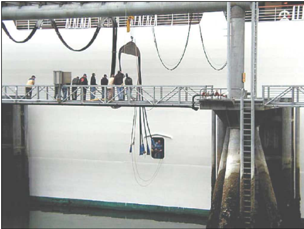
Figure IV-3: Steel Gantry Festooning System at Juneau, Alaska
