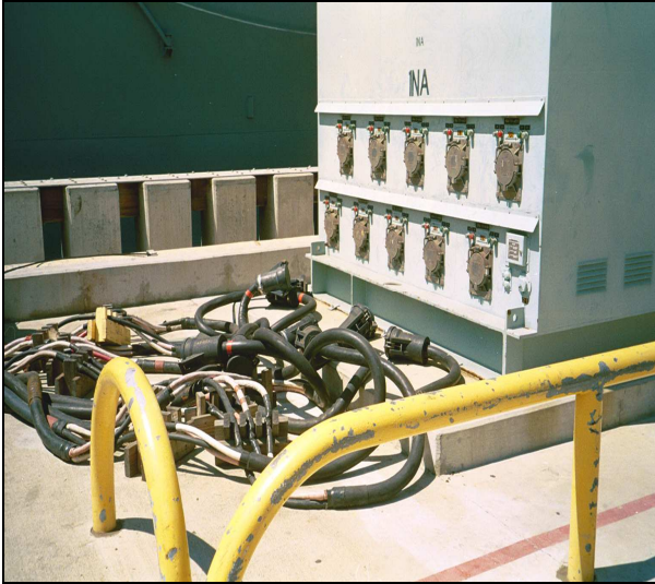
Figure IV-10: Plugs stored at a substation at the San Diego Naval Station
