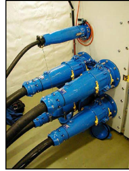
Figure IV-5: Cables Connected to an Electrical Cabinet on a Princess Cruises Ship
