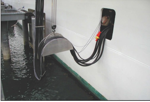
Figure IV-4: Cables Entering a Princess Cruises Ship
