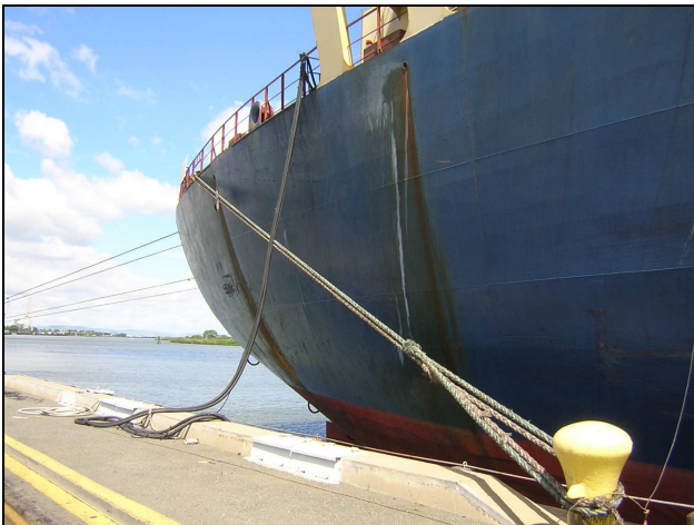
Figure IV-7: Shore-side power connection at the USS POSCO facility in Pittsburg, CA
