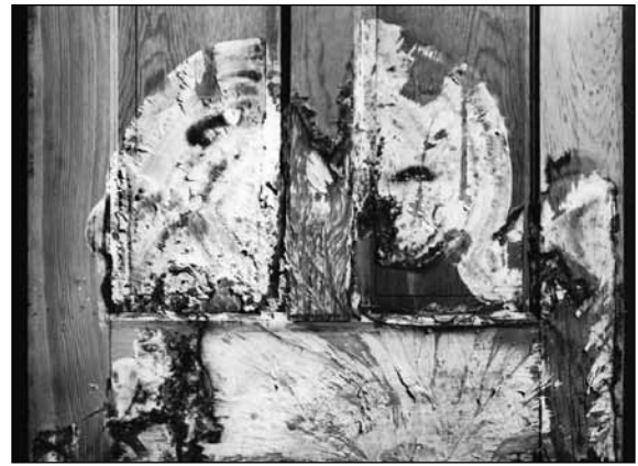
Figure 14-4. Mycelial fans on a wood door.
