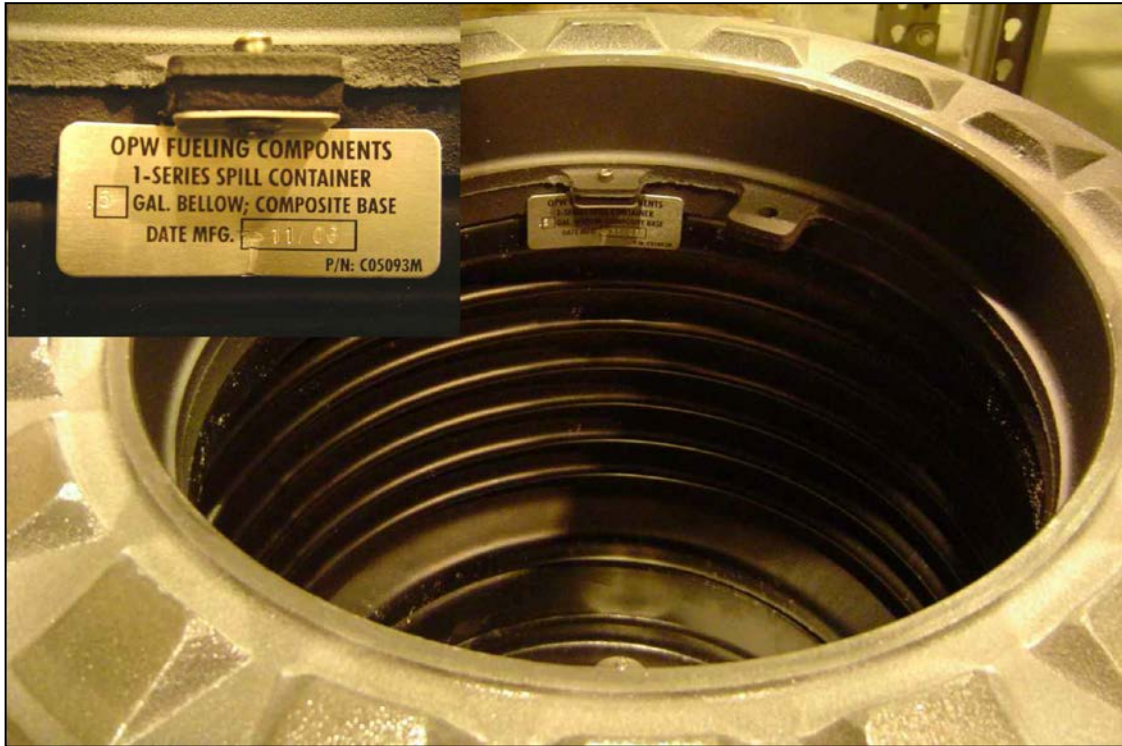
Figure 1-1 Direct Bury Spill Container OPW 1-Series (GAS/E85)
